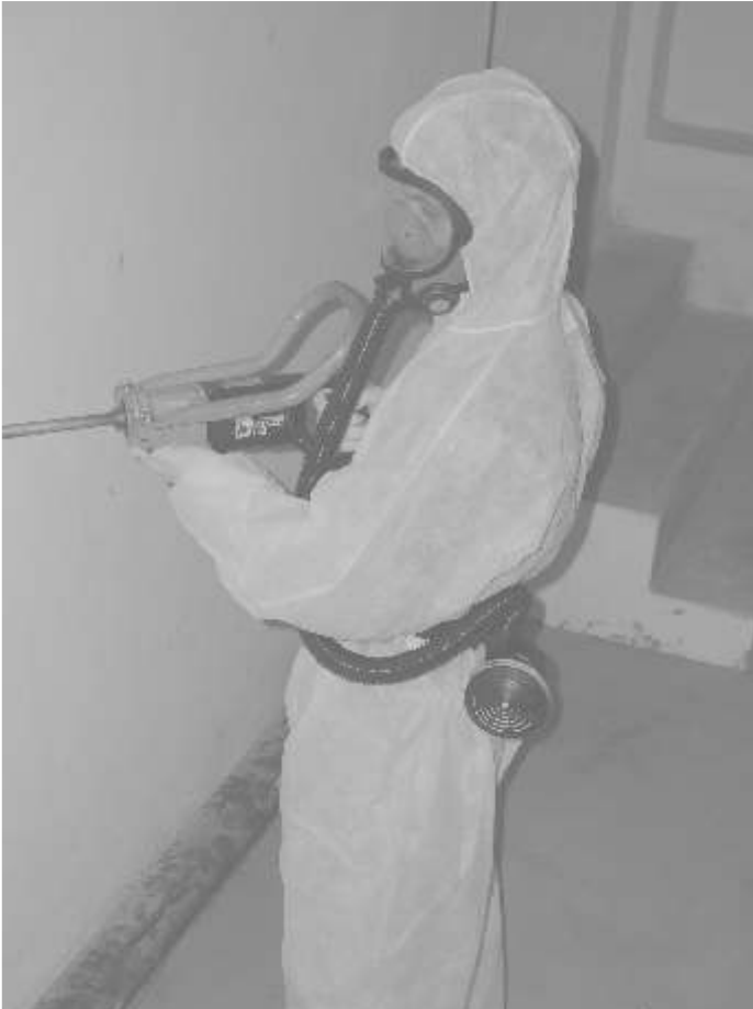
CA Asbest unit worn on the belt and connected to the mask by a hose
